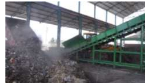
Kanpur Integrated Waste Management Facility
