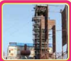
TG Building, Boiler & ESP Structure view at Nakodar
