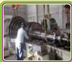
Erection of Turbine at Nakodar
