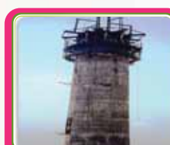
Chimney Shell Construction at Kanpur
