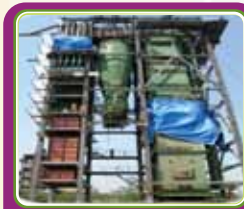
Erection of Boiler Pressure parts at Nakodar
