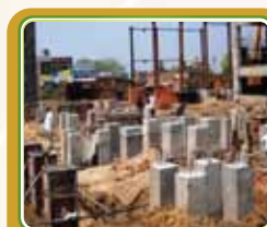
Switchyard Foundations & Erection of ESP Structure at Morinda
