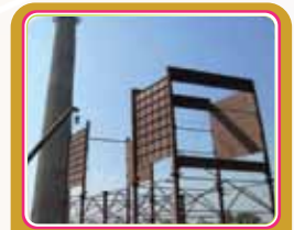
Erection of ESP & Chimney view at Nakodar
