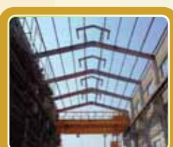
Erection of EOT Crane in TG Building at Kanpur
