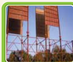
Erection of ESP Structure at Fazilka
