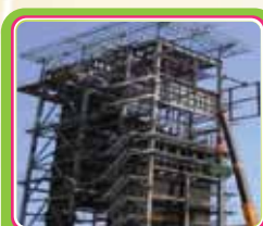
Erection of Boiler Pressure parts at Morinda
