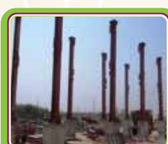
Erection of ESP Structure Columns at Kanpur
