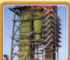
Erection of Boiler parts at Fazilka
