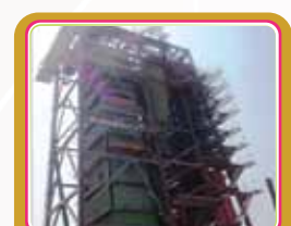
Erection of Boiler Pressure parts at Kanpur
