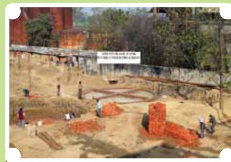
TG Condensate Storage tank
