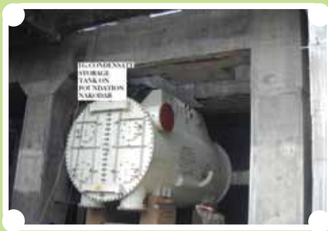
TG Condensate Storage tank
